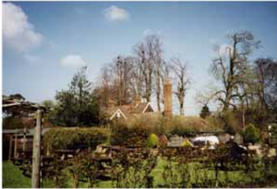
Fig 20: Peach Cottage extension and chimney
