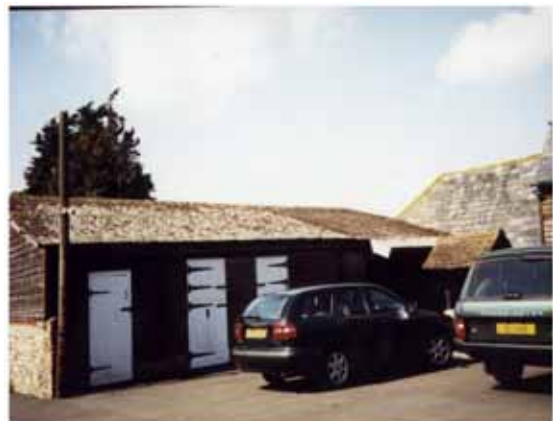
Fig 3: Stable Block, Holywell Farm
