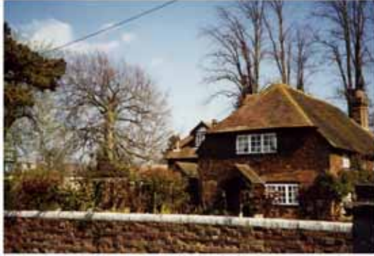
Fig 15: Brick walling with white painted brick capping
