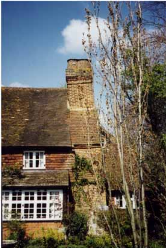
Fig 6: Chimney stack, Holywell Farmhouse
