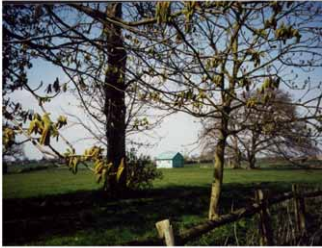
Fig 23: Timber weatherboarded pavilion, adjacent to Holywell Park
