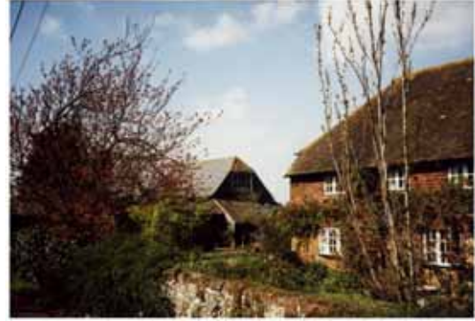
Fig 16: Brick and flint wall, Holywell Farm
